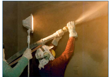
Gunite Installation
